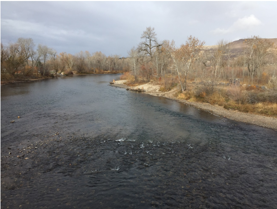
December 9, 2016 - View from Eckert Bridge of completed Engineered Log Jams, river < 1,000 cfs
