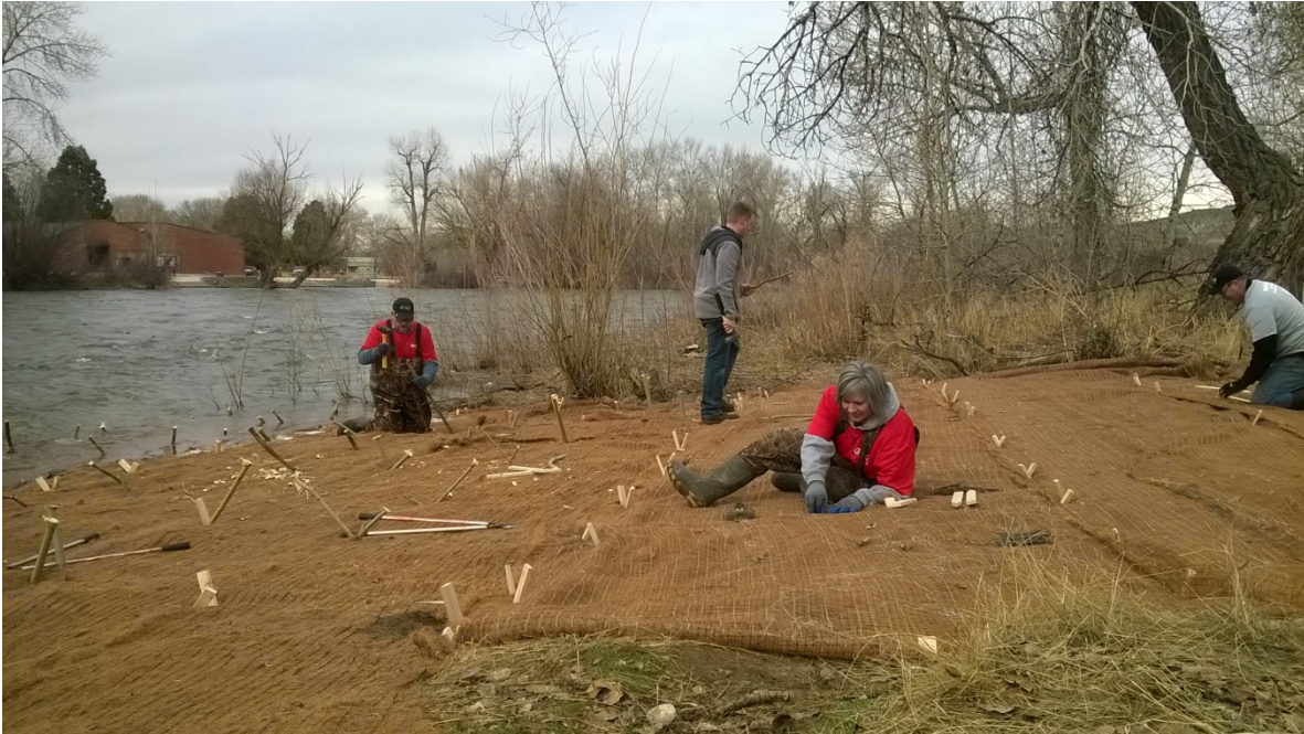
January 22, 2017 - Coconut mats being staked down to protect top soil from high water.
