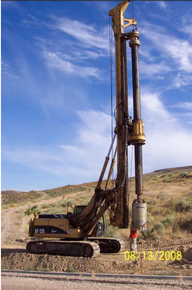
Landfill Gas Well-drilling Rig.
