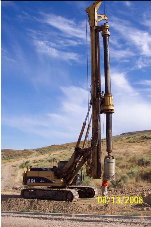
Landfill Gas Well-drilling Rig.
