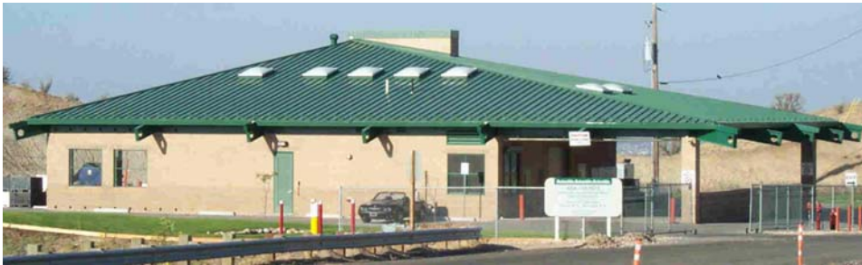
Ada County's Household Hazardous Materials Collection Facility
