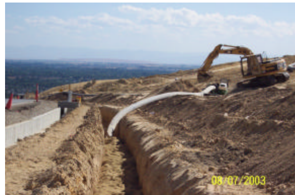
Figure 8 Installation of Header Pipe
