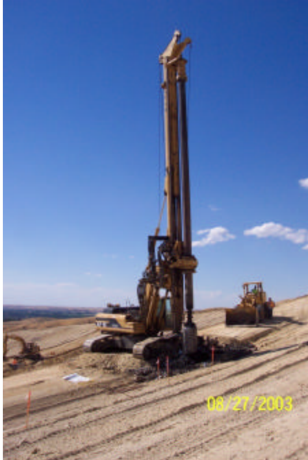
Figure 9 Landfill Gas Drill Rig
