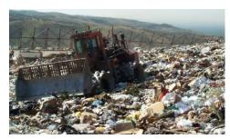
compaction of waste material. Efficient compaction provides for maximum placement of waste within the smallest space possible. Compaction ensures less airspace is lost to voids or pockets within the landfill.
