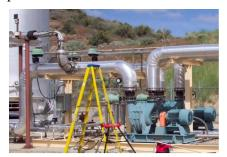
landfill with a vacuum device attached. Within the landfill, the pipes must be perforated to create the path for the gas. By adjusting the vacuum on the collection system, areas of low pressure/low concentration are created and become the preferred pathways for the gas. Connect the collection system to a destruction device, such as a flare or internal combustion engine, and the landfill gas with its odorous components are destroyed.
