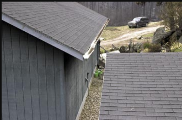
A home with a clean, non-flammable roof and gravel at the foundation.
