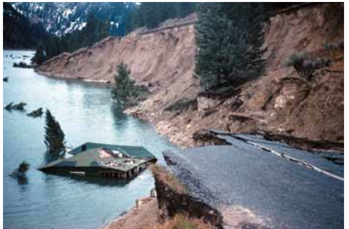
The largest historical earthquake in the Intermountain Seismic Belt was the August 1959 magnitude 7.3 Hebgen Lake earthquake in Montana. Landslides triggered by the shaking submerged Highway 287 (USGS photo).
