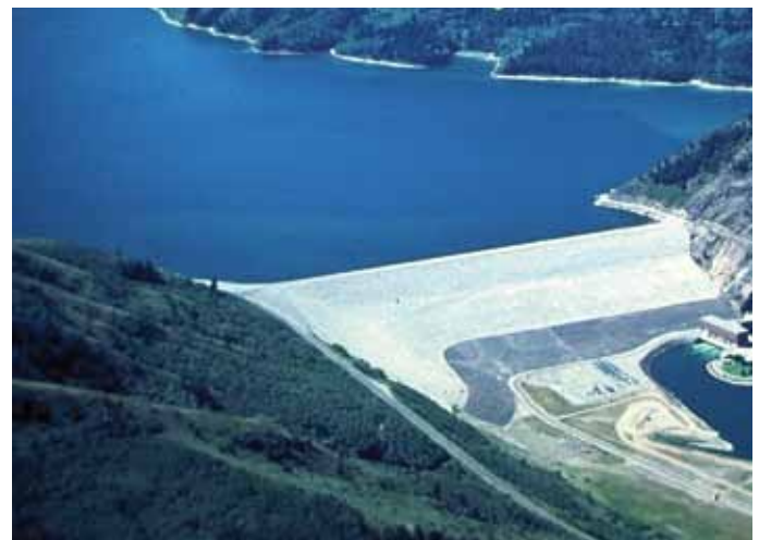
View of the Palisades Dam and Reservoir. Constructed in 1957, the Palisades Dam is 240 feet high and 2100 feet long. It dams the South Fork of the Snake River 18 miles west of the Idaho-Wyoming border. The reservoir is operated to supply about 670,000 acres of irrigated land in southern Idaho, generate about 177,000 kilowatts of hydroelectric power, and control floods. The trace of the Grand Valley fault zone is about 2.5 miles northeast of the dam (Bonneville Power Administration photo).
