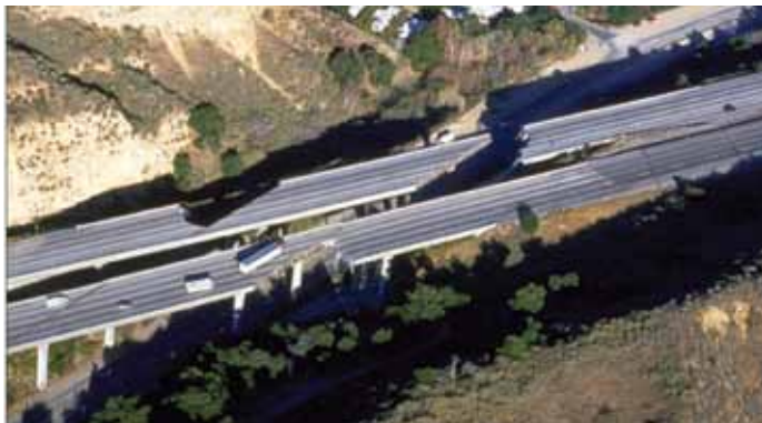
Damage to Interstate 5 in 1994 Northridge, California, earthquake. (Photo courtesy of FEMA)
