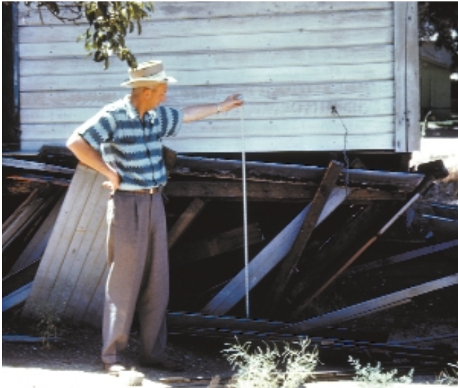
Failure of wood frame dwelling. A post-and-pier foundation with a cripple wall, Kern County, Calif.
