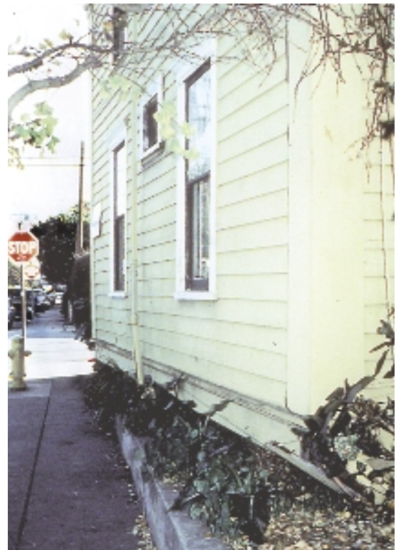
Cripple wall foundation failure, Northridge, Calif.
