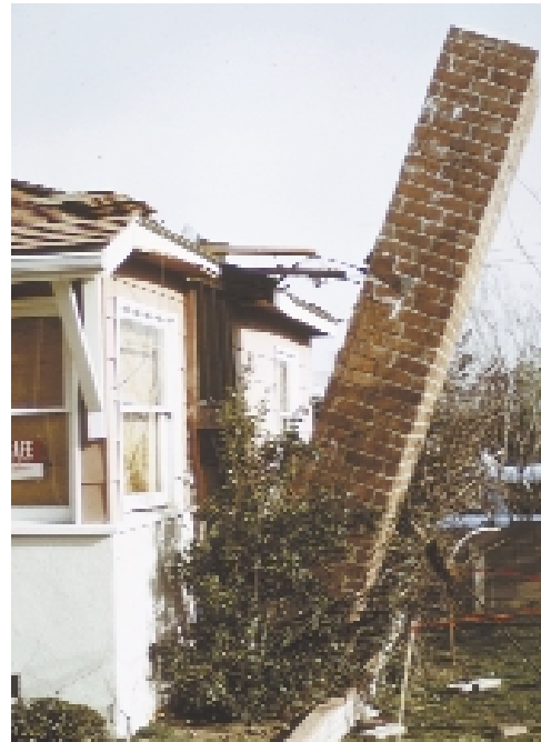
Chimney damage, San Fernando, Calif.
