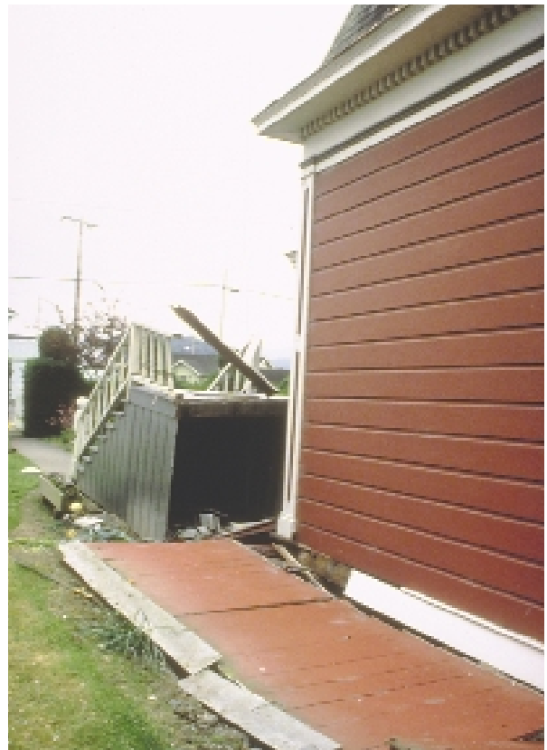
Post-and-pier with cripple wall foundation failure, Ferndale, Calif.
