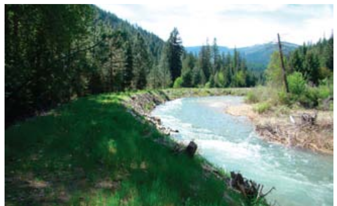
Figure 7 : Pine Creek Levee, Pinehurst, Idaho. Photo courtesy of USACE Seattle District
