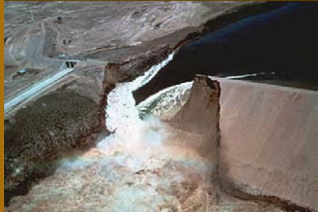
Figure 3 :Teton Dam Failure
