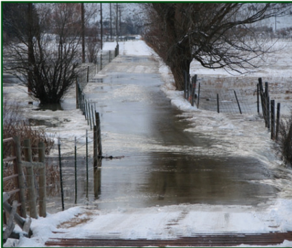
Figure 10 : County road in Lemhi County flooding due to ice jam on the Salmon River in January 2010
