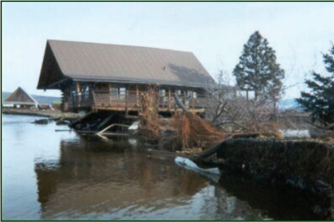
Figure 34 : Flood damaged home from 1997 flood.
