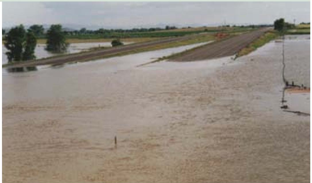
Figure 22 : June, 1997 Snake River flooding of Interstate 15 between Blackfoot and Shelley.
