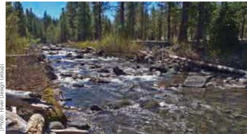
Wychus Creek, OR. A diversion structure that was a fish passage barrier (upper photo) was upgraded to provide fish passage by creating a "rock ramp" or engineered riffle (lower photo).
