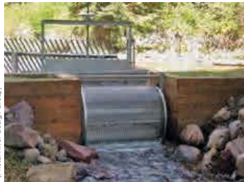
Morell Creek, OR. Both rotary drum (left) and flat panel screens were used on different diversions to prevent fish entrainment.
