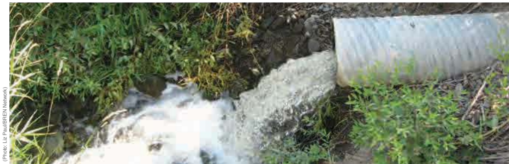
Outfall from CB River Spring Ranch wetland complex near Parma. Wetland systems can be used to clean water. The wetland complex at CB Spring Ranch receives irrigation drain water from over 1,200 acres of upstream farmland.
