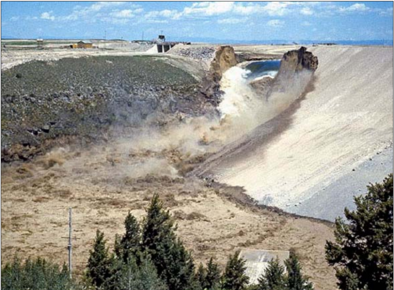
Figure 7-2. Teton Dam Failure, 1976
