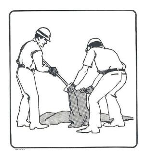
For large-scale operations filling sandbags can be expedited by using bag-holding racks, metals or plastic funnels, and power loading equipment. However the special equipment required is not always available during an emergency. Bags should not be filled more than half full or less than one third of their capacity.
