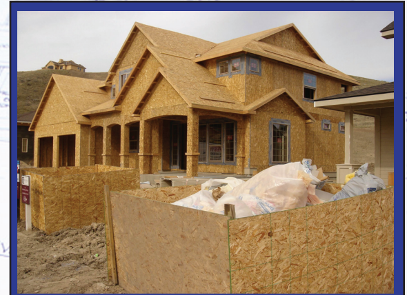
Example of Good Debris Collection
